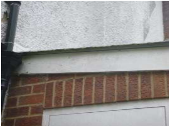
9. The tight barge board and tightly fitted corrugated roof on the garage.
