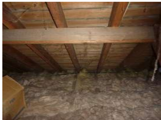
12. Eaves filled with fibreglass.
