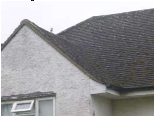
5. The intact mortar under the verge tiles on the rear gable end.
