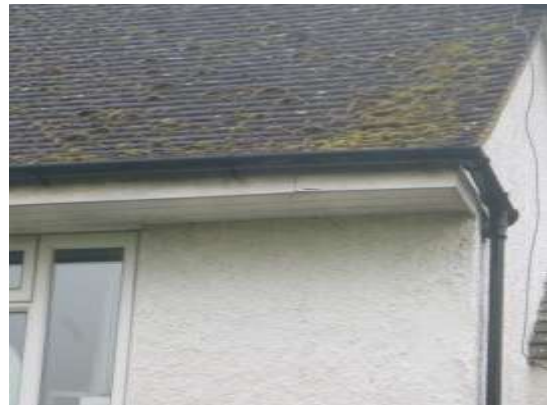
6. The tight soffit box.
