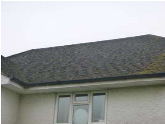
3. Tightly fitted roof tiles and intact mortar under the ridge tiles.
