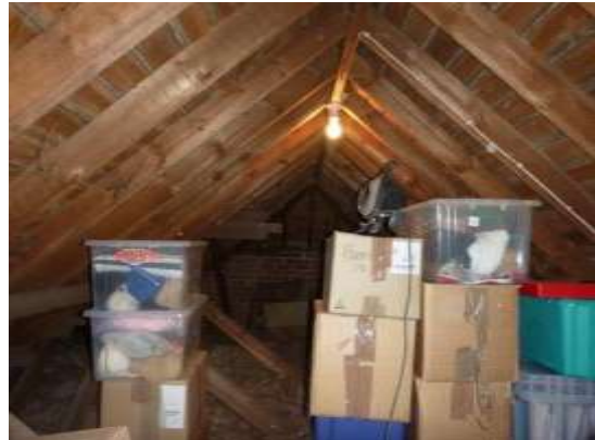
10. Fibreglass which was fitted between the joists.
