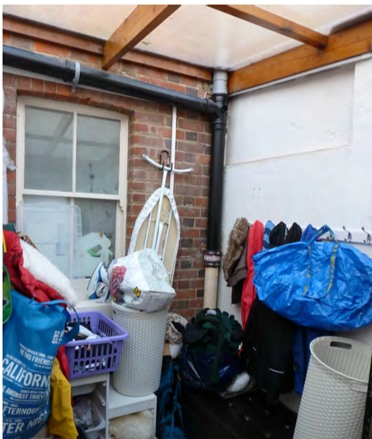
Fig.3: Interior view of existing utility room
