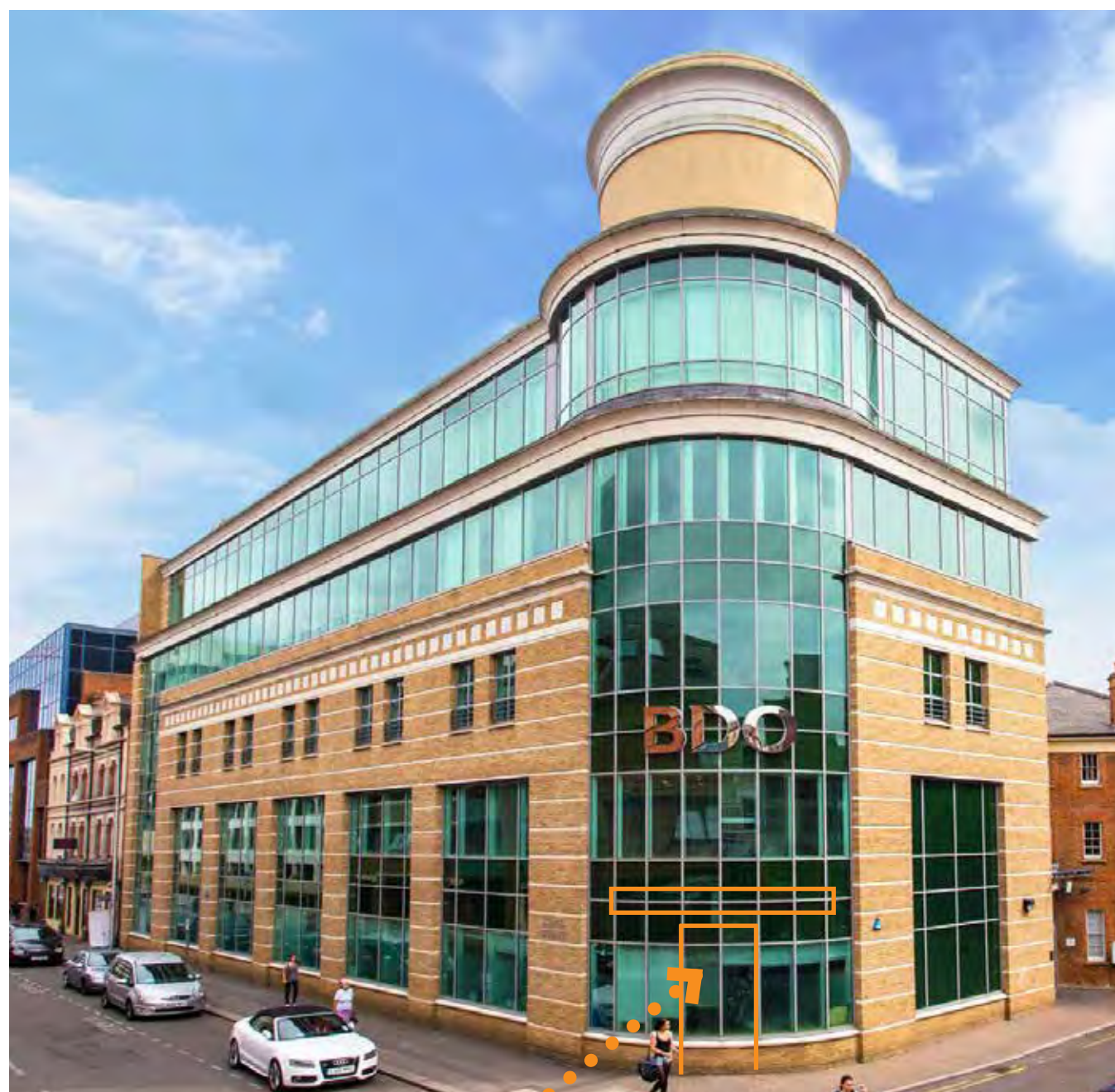
New main entrance with canopy above
