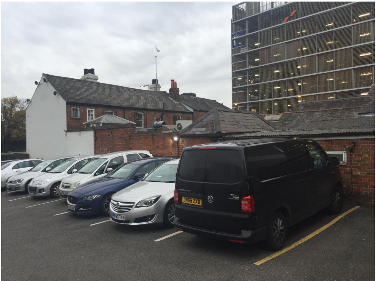
Fig 4: West Elevation with multi-storey car park in the background
