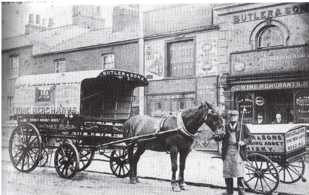
Fig 7: Butler's Wine Vaults, 1907
