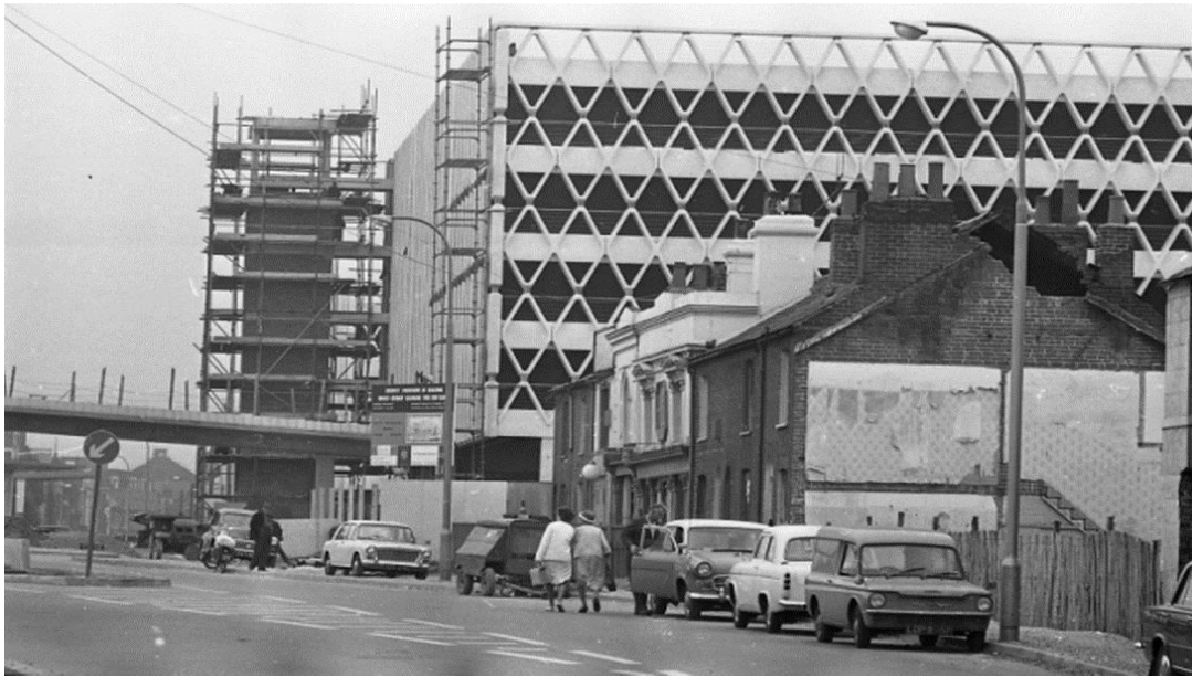
Fig 8: Construction of Chatham Street Car Park, 1968
