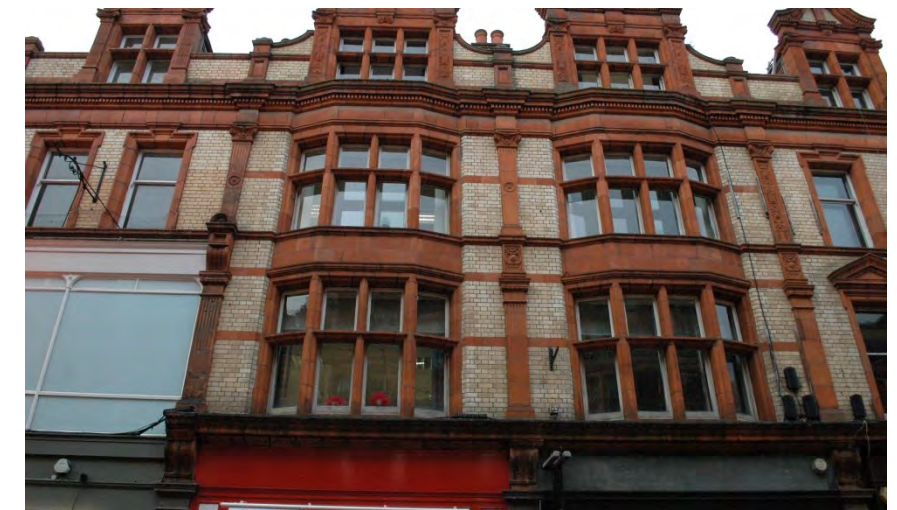
Plate 15: Front façade of 17 Queen Victoria Street
