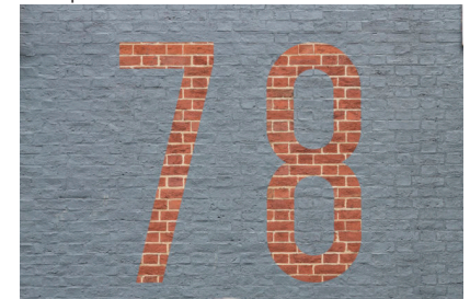
Building numbering in brick work
