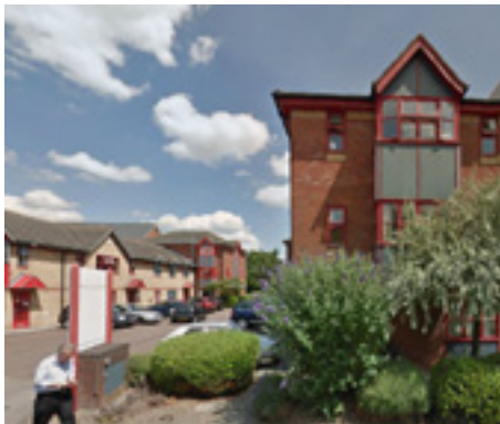
3 Storey Windsor Court - adjacent to the site
