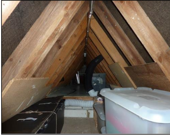
Photograph 7: Internal roof void.
