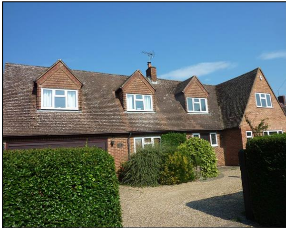
Photograph 1: Front of house, south facing.
