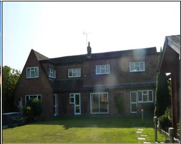
Photograph 2: The rear of the house, north facing.
