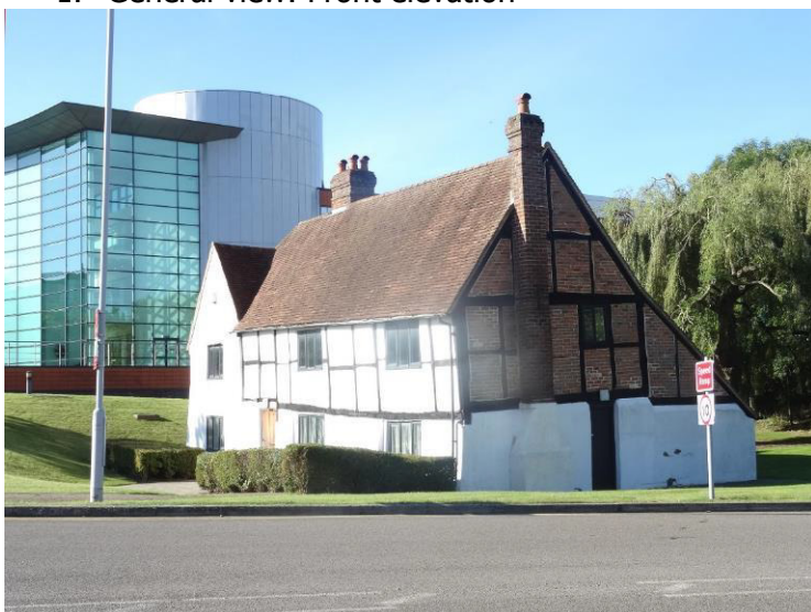
2. General view: Front and north elevations
