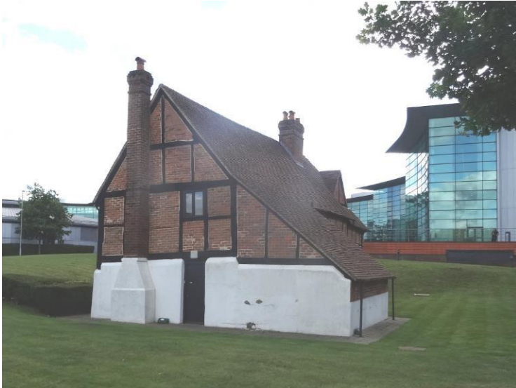
3. General view: North and rear elevations and Reading International Business Park.
