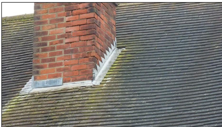
Figure 7 – roof showing clay tiles and ridge section on the rear elevation
