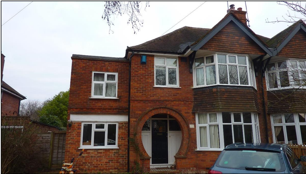
Figure 2 - Front elevation of 154 St Peters Avenue
