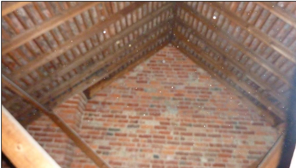
Figure 4 – showing interior of roof void at 154 St Peters Road
