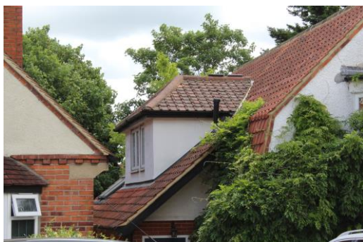
Existing dormer & Roof to adjacent premises
