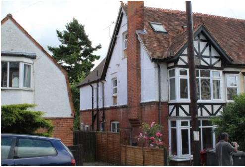
Side wall to no 16 St Annes Road
