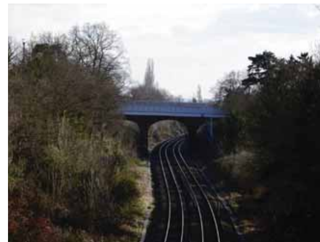
Figure 10: Bath Road Overbridge seen from Tilehurst Road
