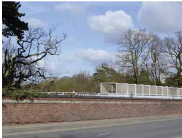
Figure 9: Detail of low mileage parapet showing the modern footbridge in the background
