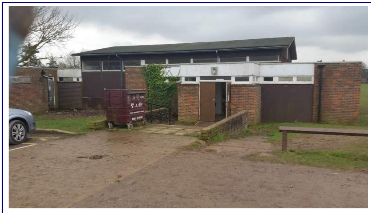
General view of the site (facing west). Further Photos are included within Appendix B.
