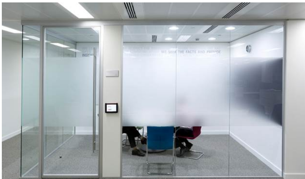
Photograph of typical glazed acoustic screen
