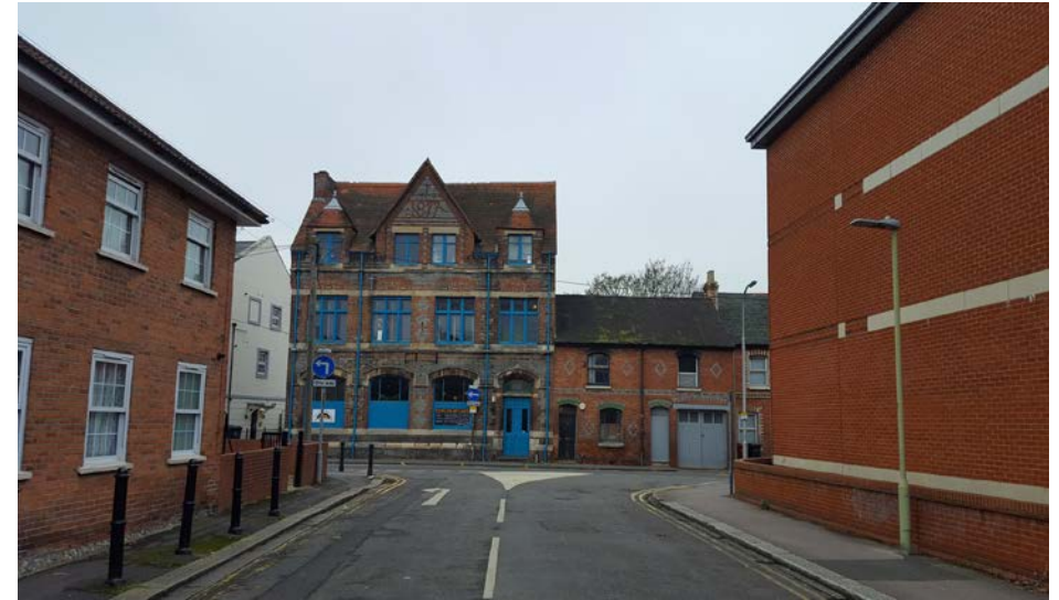
Photo: View of 30 Silver Street showing grey feature brickwork
