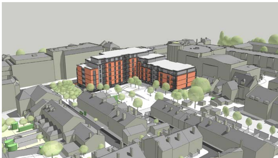
Aerial view from southwest
