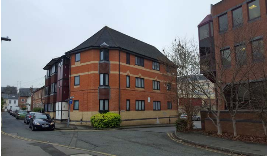
Photo: View of 1-14 Priors Court from north
