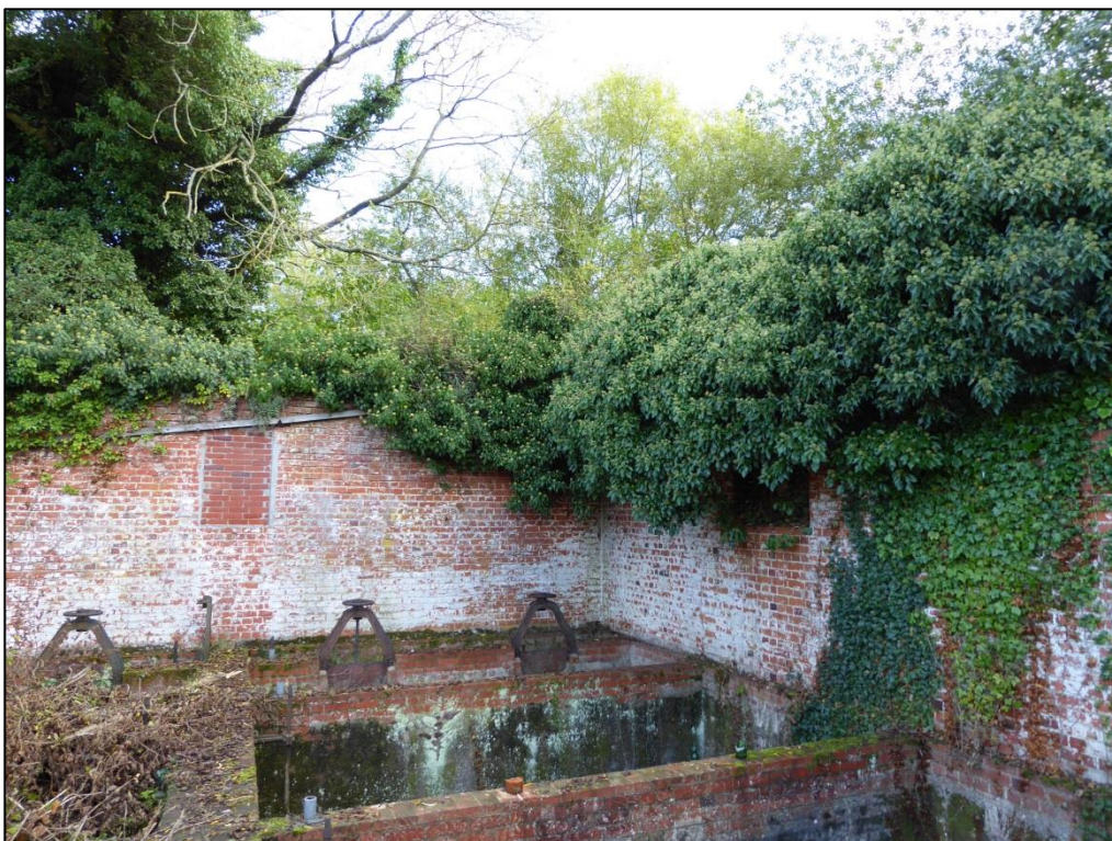
Figure 4. Interior of the former wire mill, Southcote Mill. 16.09.15.
