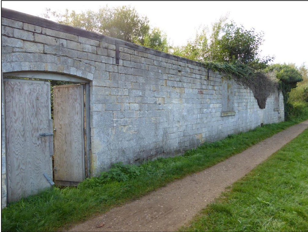
Figure 3. Exterior of the former wire mill, Southcote Mill. 16.09.15.
