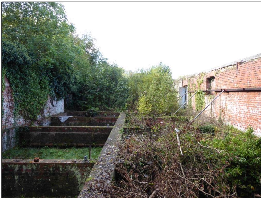
Figure 7. Interior of the wire mill, Southcote Mill. 16.09.15.
