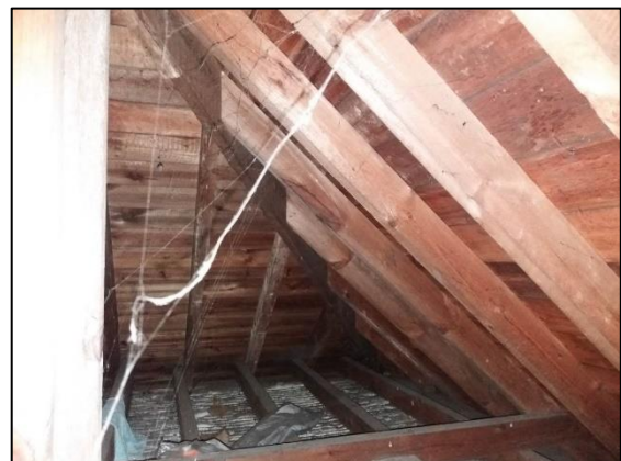
Photograph 6: Crawl space at eaves
