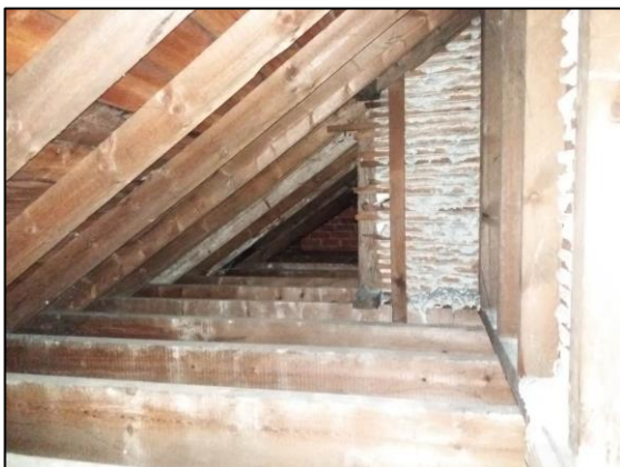
Photograph 5: Crawl space at eaves
