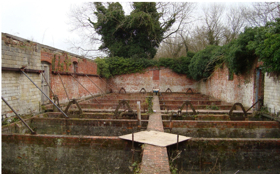
Internal view of The Wire Mill
