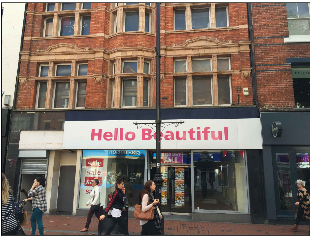
Existing shopfront photo
