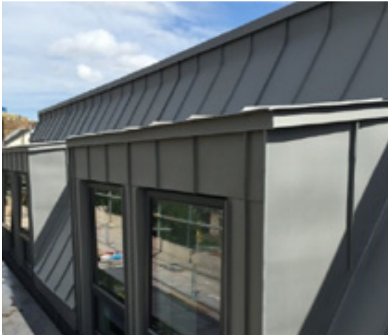
Zinc clad dormer and roof (indicative image)
