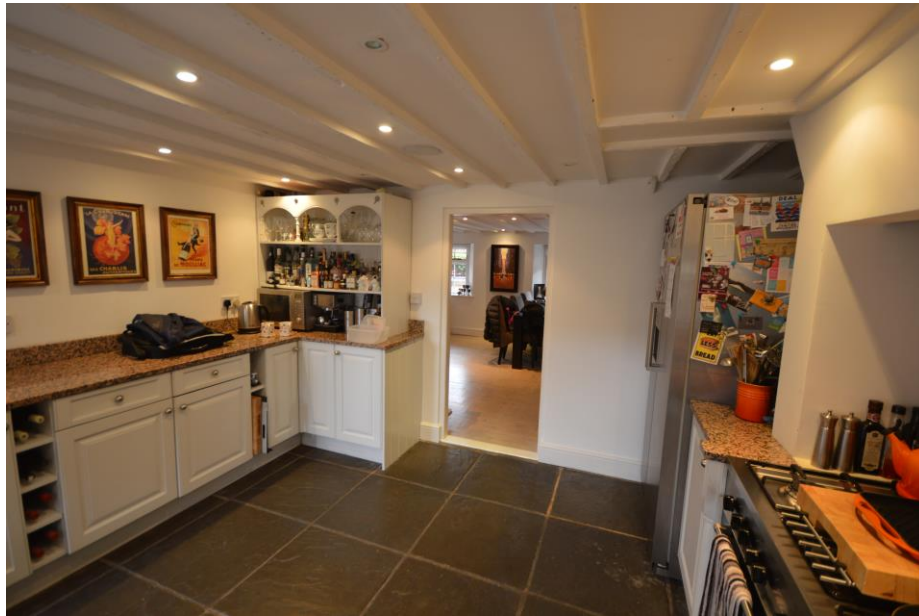
Pic.3 internal wall to be partially removed, leaving 'nibs' to either side to support structure.
