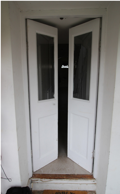
Existing rear entrance doors.
