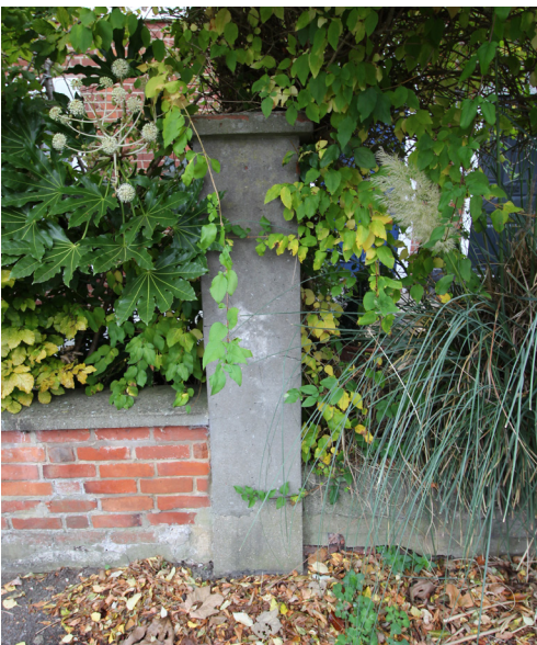
Cement rendered pillar at boundary with neighbours brick wall.
