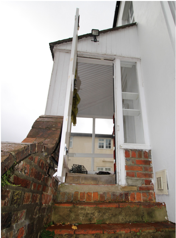
Existing conservatory approved for removal under application 162026.
