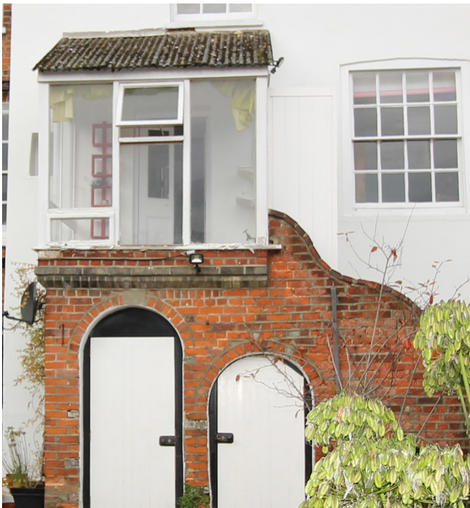
Existing rear elevation with intrusive conservatory.
