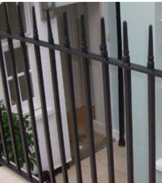
Example of spear headed railings.
