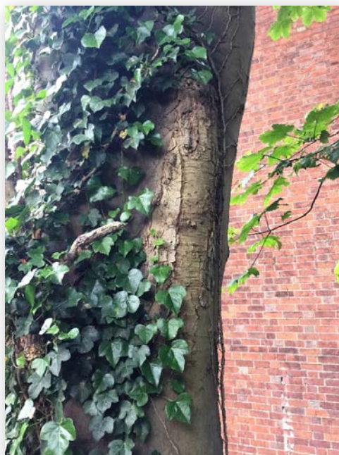
Image 3: Close up view of the west face of Tree T5's trunk showing Pronounced bulge or Rib between two stems in a compression fork
