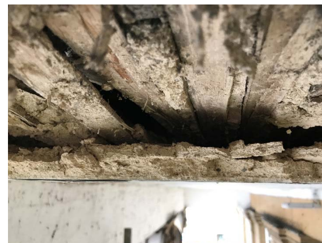
Figure 9: close up of timber laths
