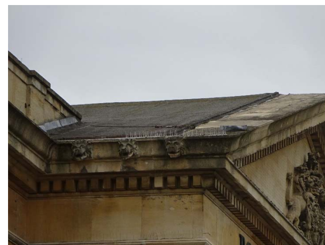
Figure 10: close up of roof covering
