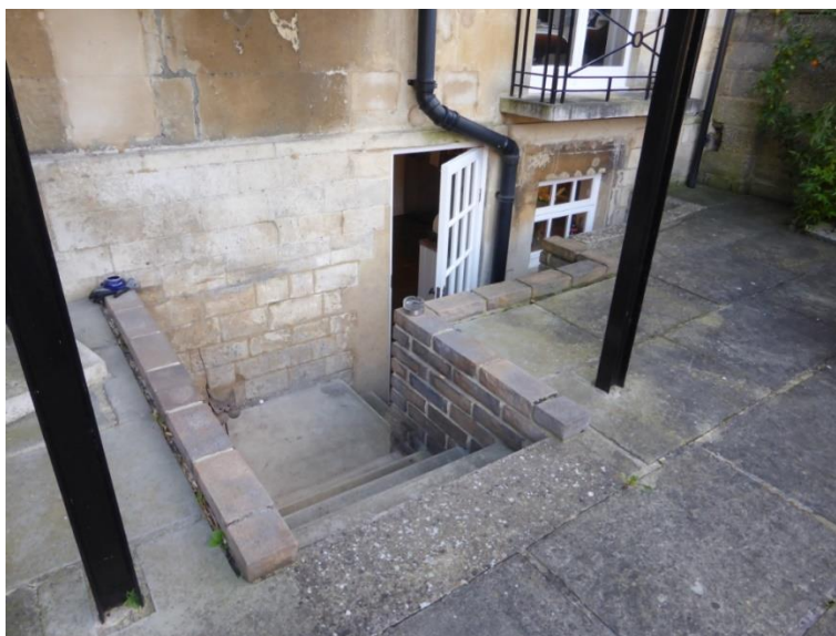
Figure 7: Modern steps and door opening to the basement from the rear garden
