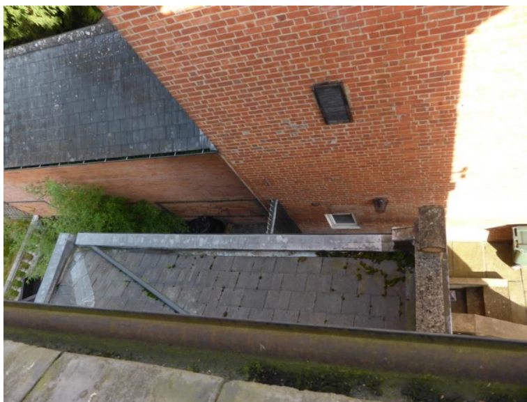
Figure 6: Shallow pitched roof and parapet of the existing side entrance
