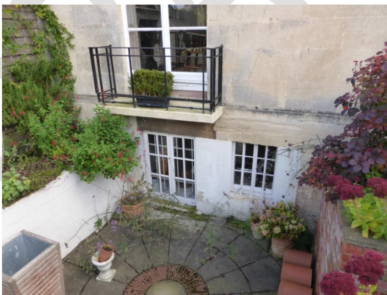
Figure 8: Arrangement of windows along the rear wall of the basement at No. 50 Russell Street
