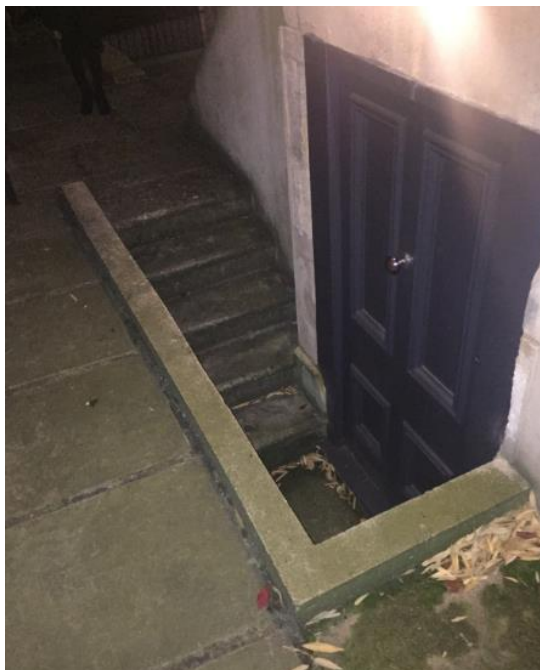
Figure 9: Servants' entrance to the basement along the north elevation
