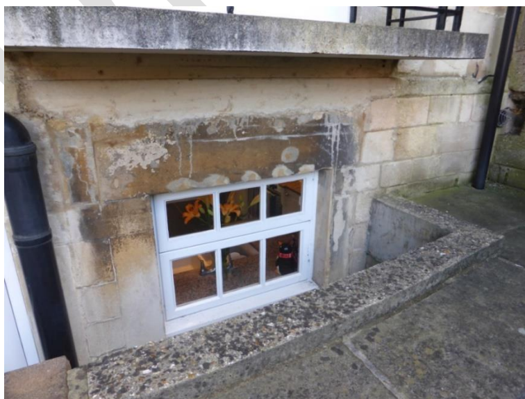
Figure 10: Modified window opening to the basement with large area of mortar infill over the lintel
