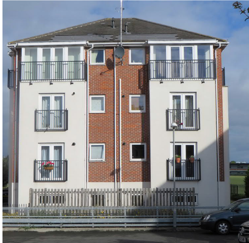
Black metal balconies at high level in Regis Park Road - cause a visual distraction
