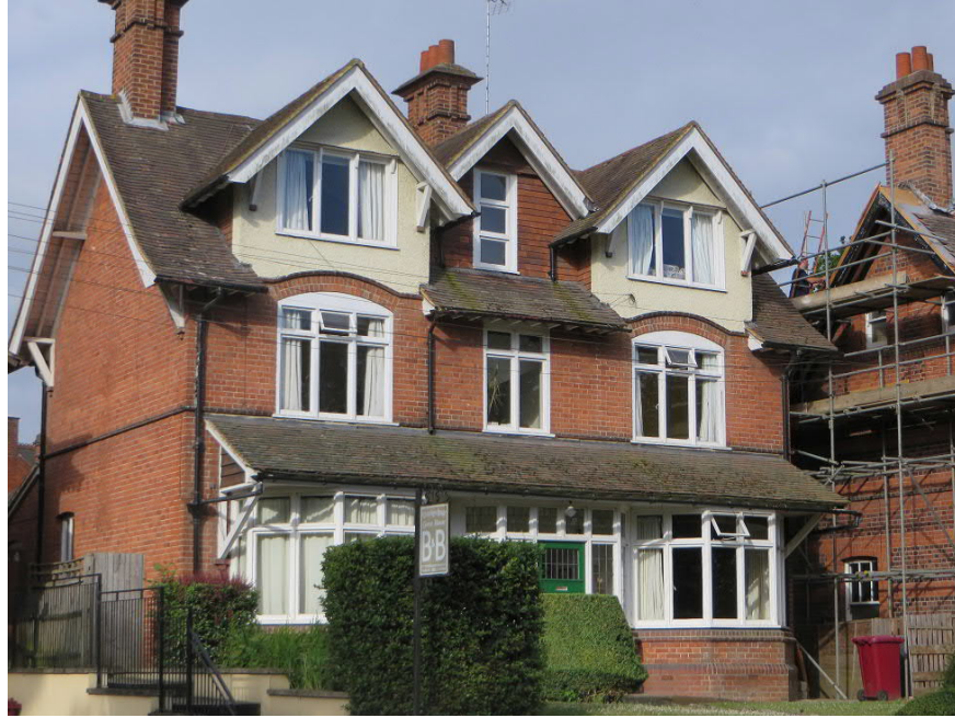
Images of Neighbouring Properties at the junction of Regis Park Road and Wokingham Road - varied application of render
