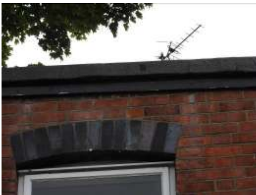
Figs. 17 & 18 Sealed eaves of the flat roof
