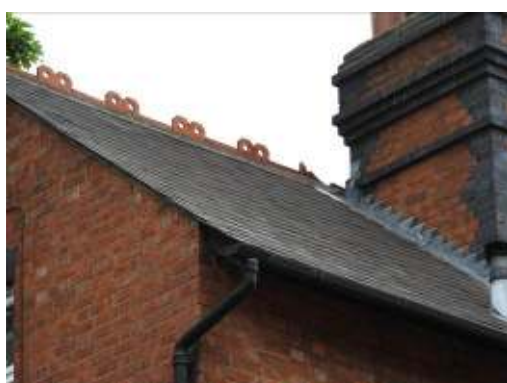
Figs. 6 & 7 Ridge and roof tiles to the south
