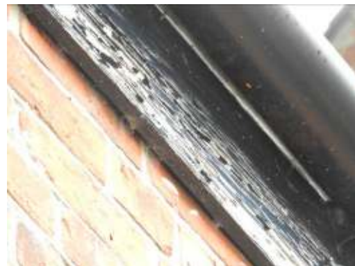
Figs. 17 & 18 Sealed eaves of the flat roof
