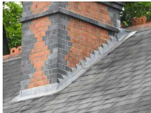
Figs. 11 & 12 Tightly moulded lead flashing
