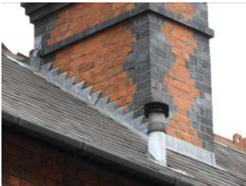
Figs. 11 & 12 Tightly moulded lead flashing
