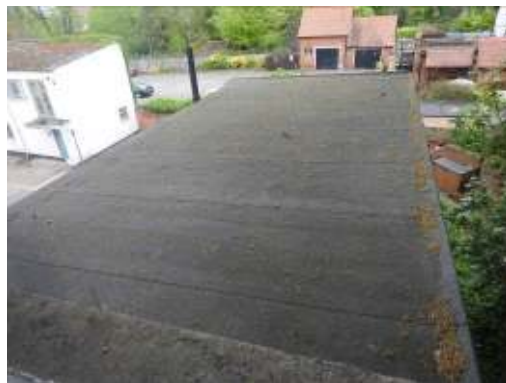
Fig. 10 Sealed flat roof
