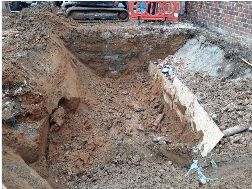
Plate 4: Photograph of completed excavation looking south west.
