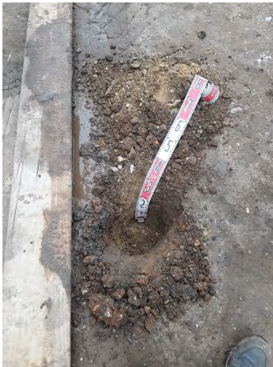
Plate 10: Hand dug pit HD04 undertaken in Plot 1, confirming 300mm of capping
