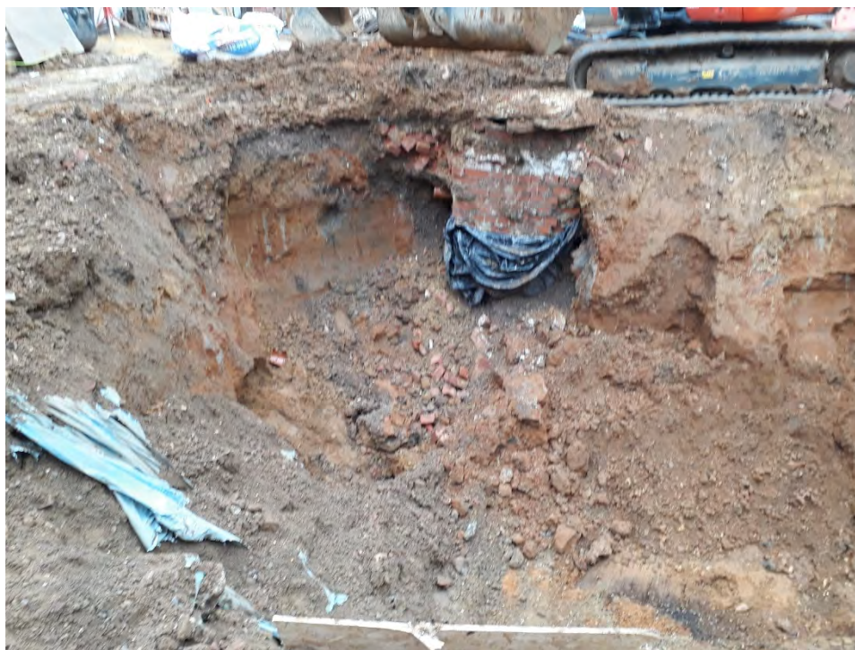
Plate 5: Photograph of excavation - Face (F3)
