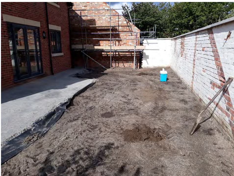
Plate 12: view of the finished garden Plot 4.
