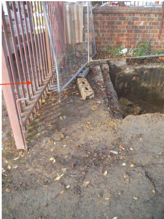
Plate 2: Photograph showing proximity of concrete chamber to site boundary and public footpath.
