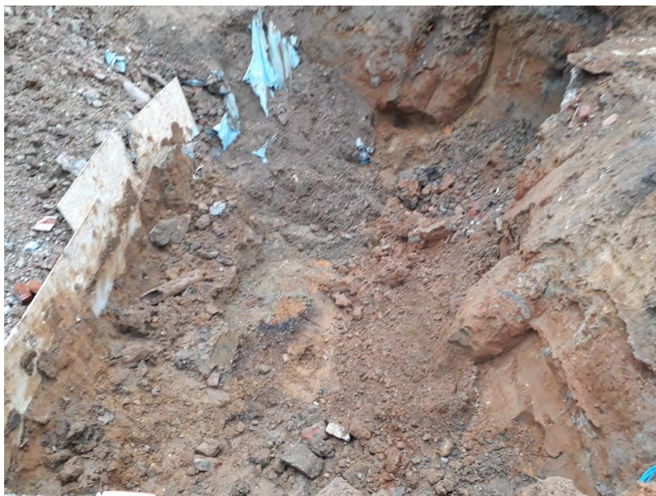
Plate 6: Photograph of excavation looking north east
