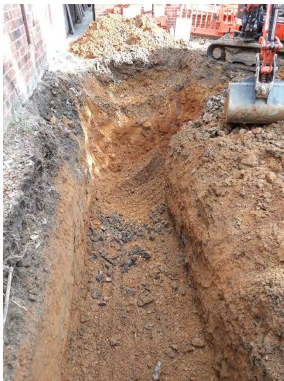
Plate 3: Excavation of contaminated soils adjacent to boundary wall looking north east.
