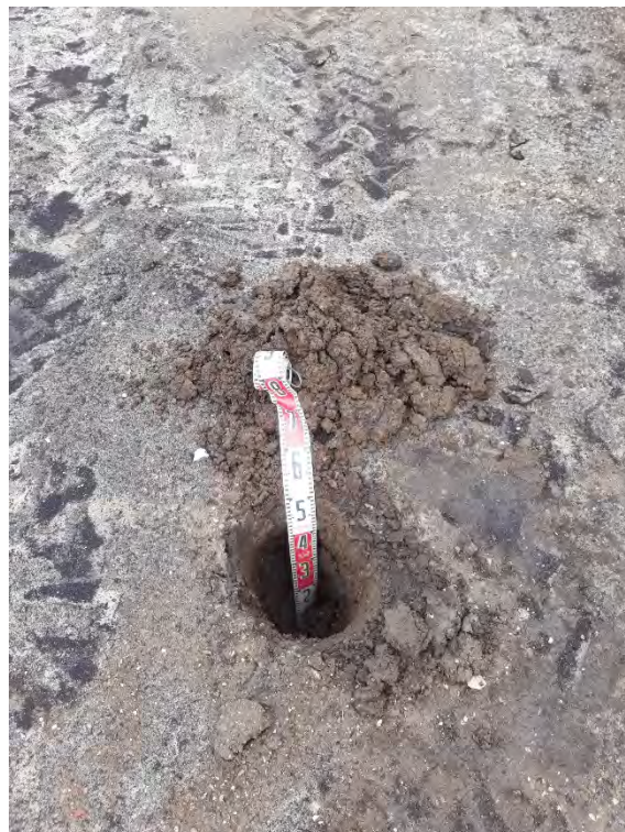
Plate 8: Hand dug pit HD02 confirming placement of 600mm of capping in Plot 4
