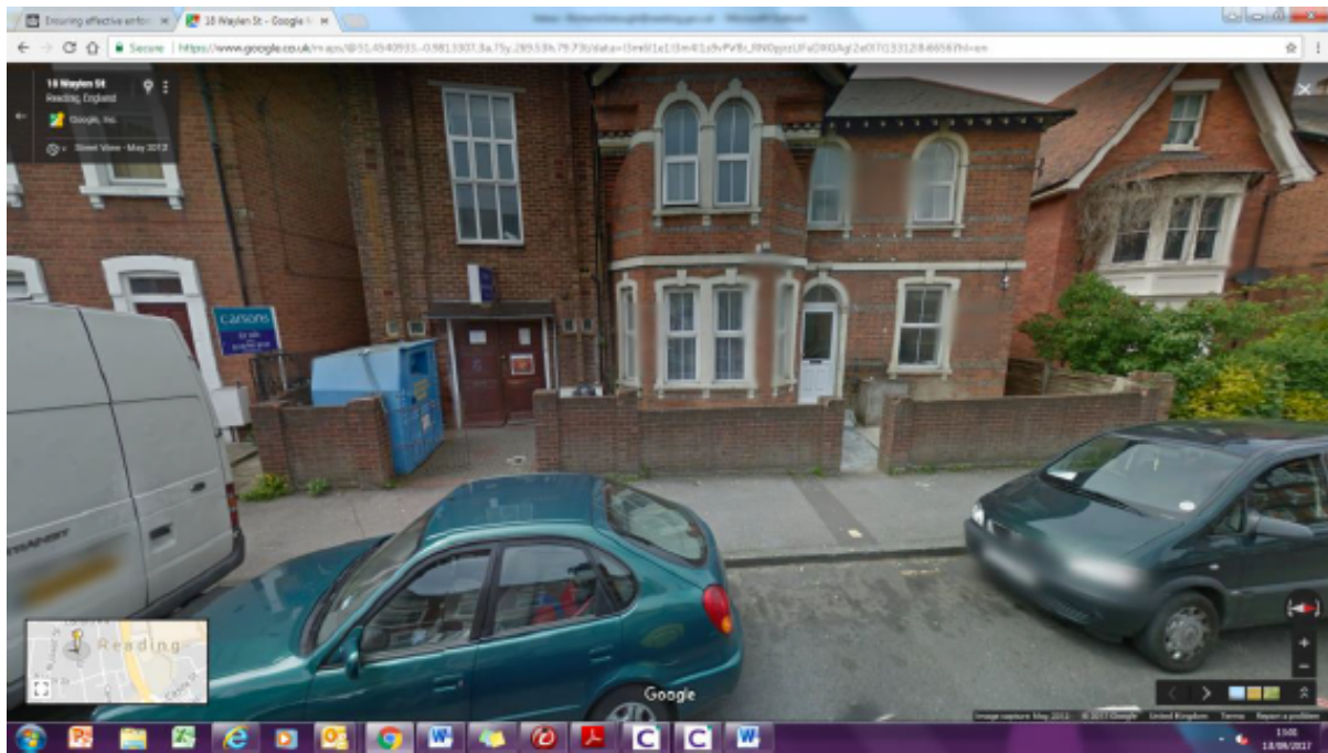
Photograph 5. Pre-existing front boundary wall.
