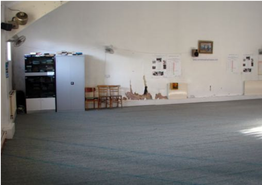
Photograph 9. Showing the gable end wall of the pre-existing building (with 20 Waylen Street towards the left).
