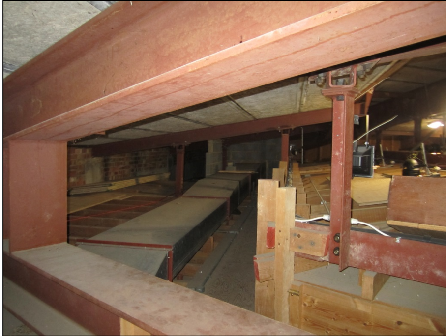
Plate 5. Roof space above brick building (Target Note 1)
