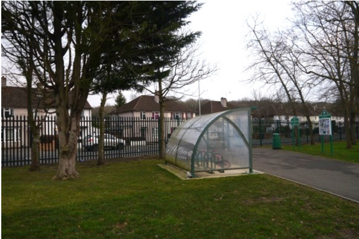
New cycle shelter constructed within the Root Protection Area of the Lawson cypress, T117.
