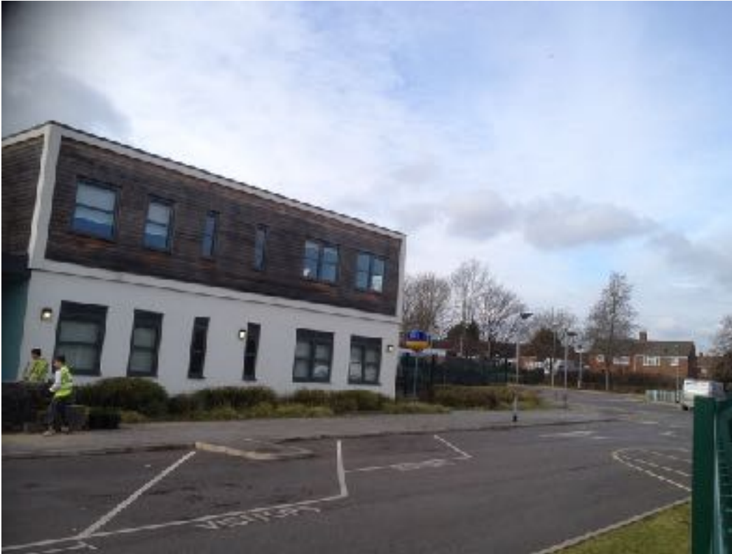
View of the two storey TVS building from the east
