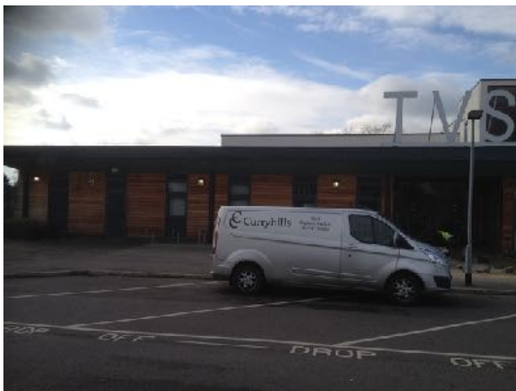
View of the single storey TVS building from the east. It is proposed to expand the two storey accommodation over the top of the single storey area.
