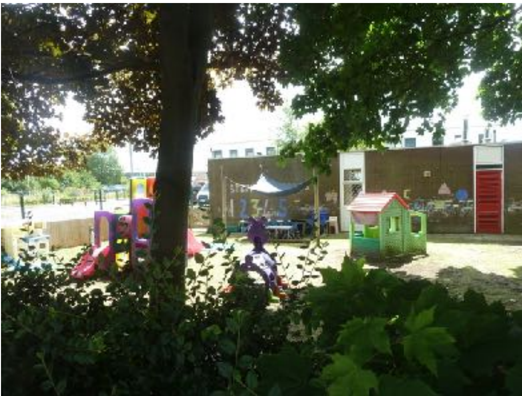
The adjoining nursery school in the former secondary school buildings viewed from the Meadway boundary north of the site
