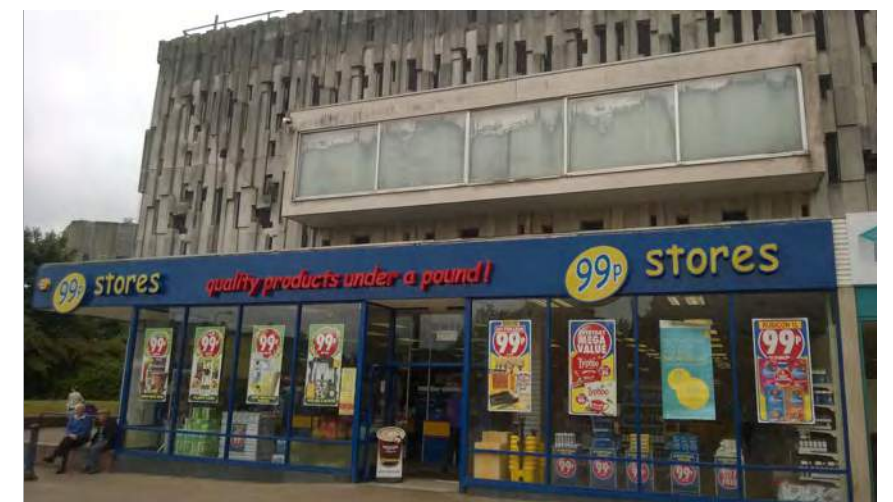
Retail Unit with Car Park above.
