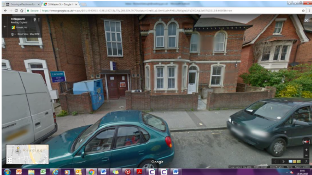
Photograph 5. Pre-existing front boundary wall.
