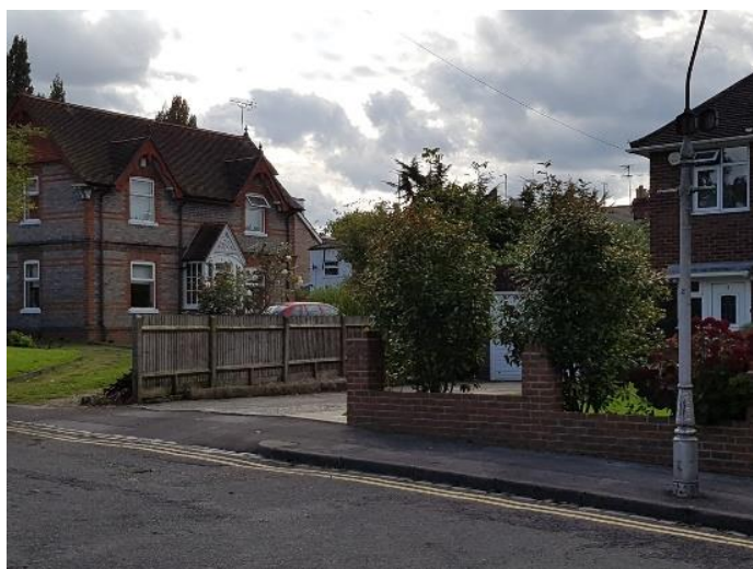
Existing Building September 2017 (at the present)
