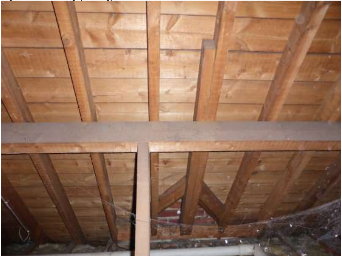
Figure 9. Tile lining (sarking) at 63 Allcroft Road. 21.7.17
