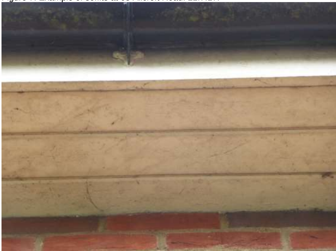
Figure 7. Example of soffits at 63 Allcroft Road. 21.7.17.
