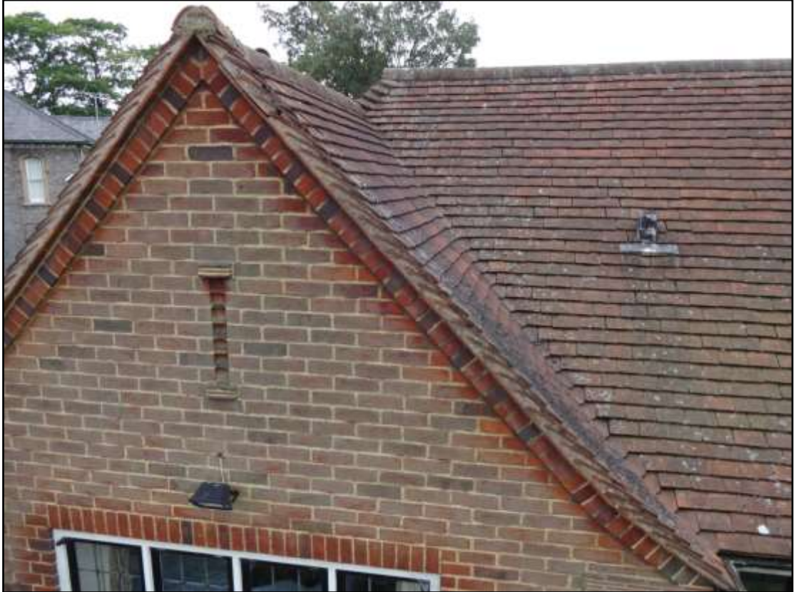
Figure 5. Gaps at front of garage roof at 63 Allcroft Road. 21.7.17
