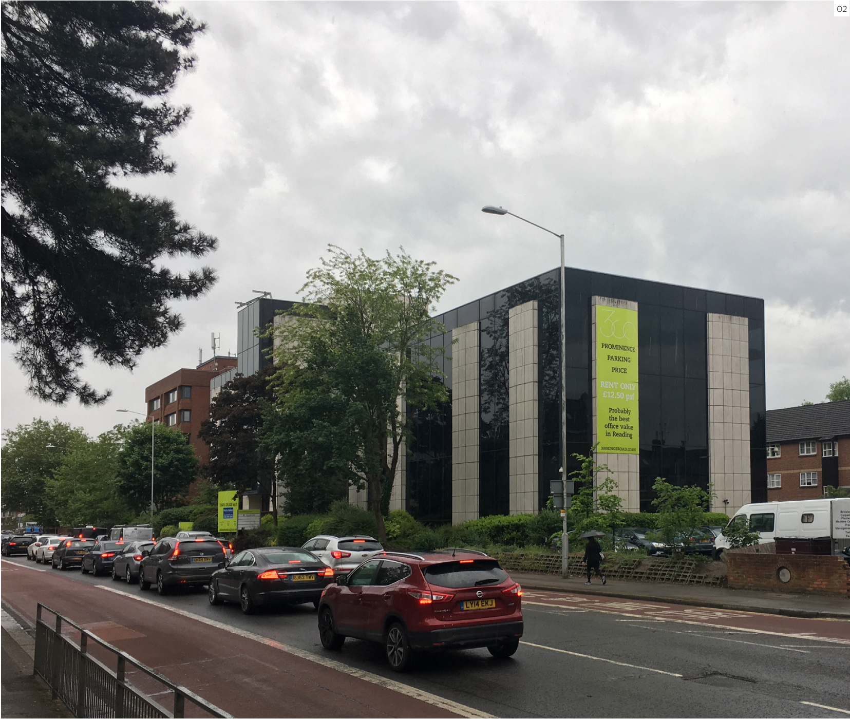
02 View looking towards Aspen house from Kings Road.
