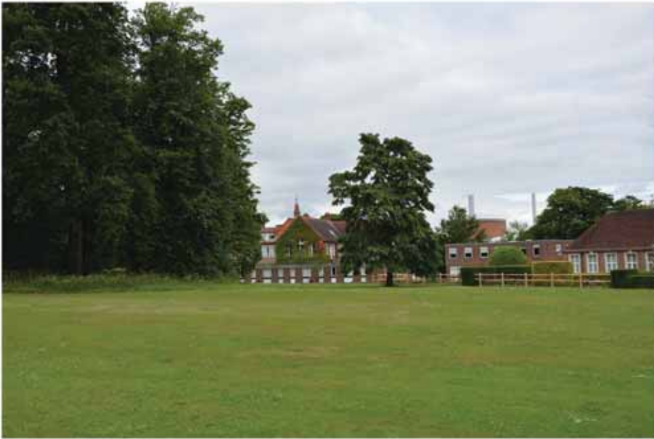
Plate 1 View north from the Site showing part of Grove House
