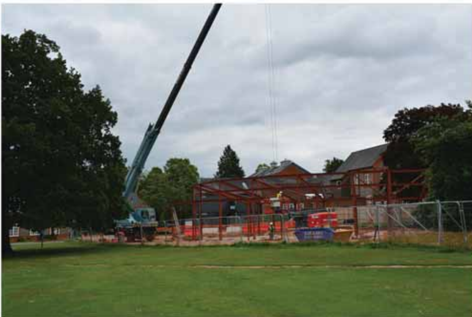
Plate 3 Construction works ongoing on new Media Centre, Grade II Listed Science Block beyond
