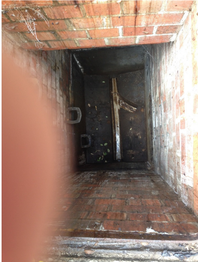
MH F5, Last Foul manhole onsite
