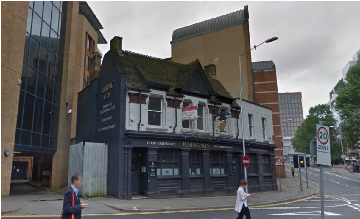
Figure 1 – Building to be demolished
