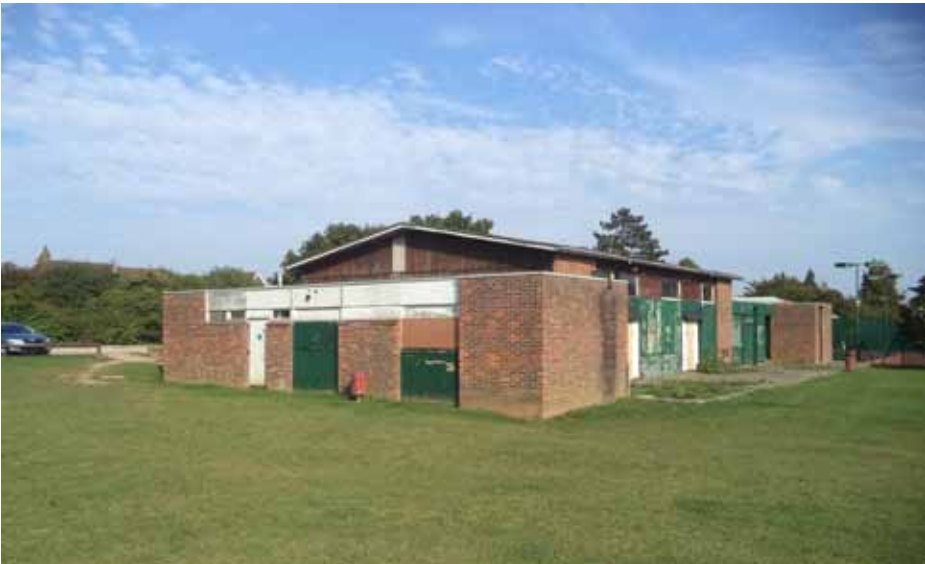
3. Image showing the existing Mapledurham Pavilion
