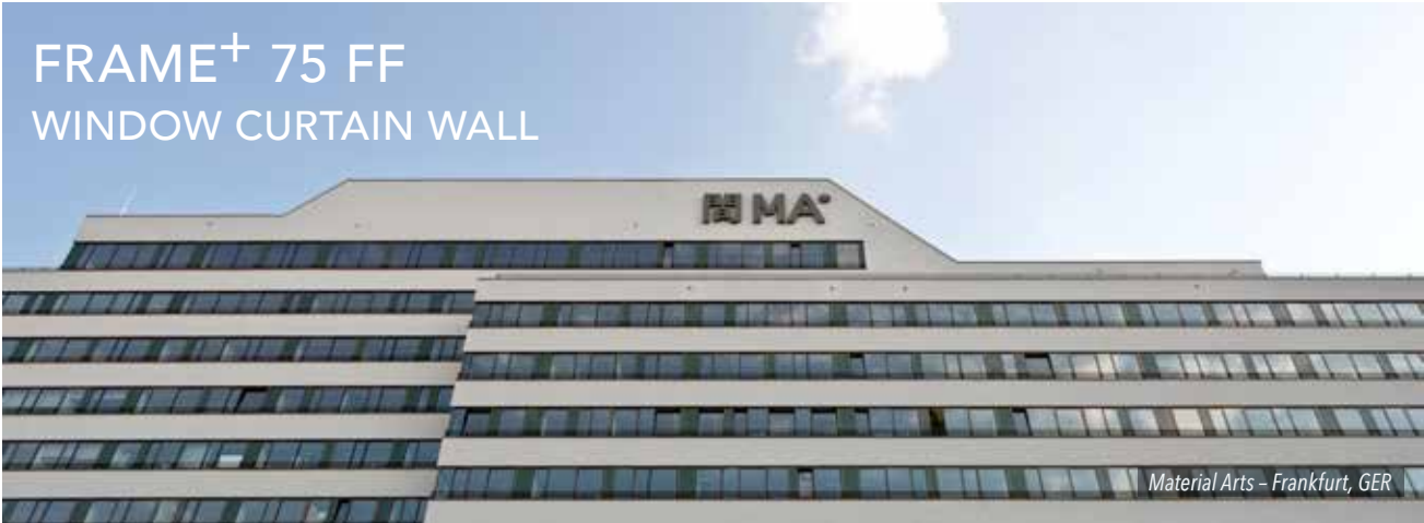
The version FRAME+ 75 FF offers additional advantages of this trendsetting window technology, such as a slim-line mullion-transom design model featuring elevation widths of only 50 mm, and an U_f value of up to 0.98 \text{ W/(m}^2\text{K)} .
