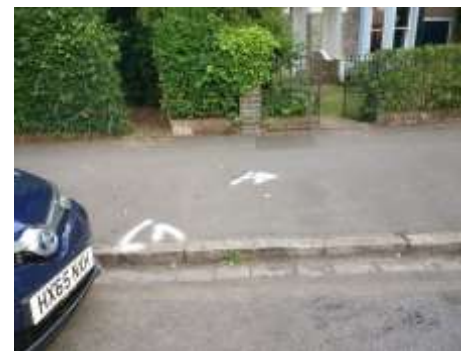
Dropped kerb to highway
