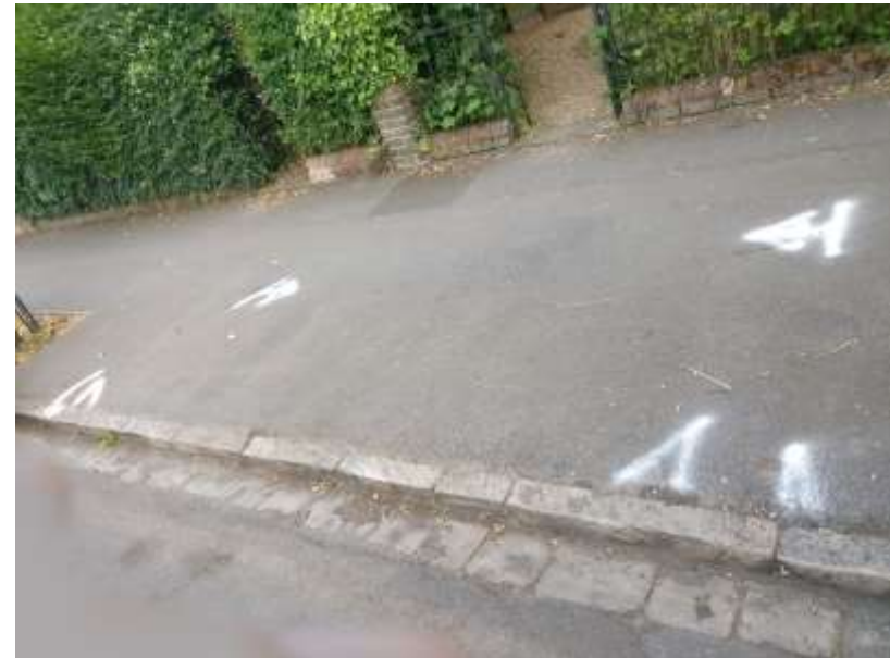
Area of dropped kerb marked out
