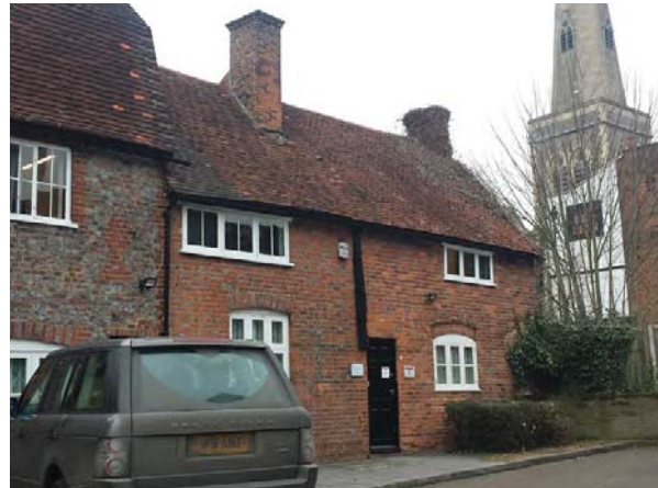
View of residential surrounding brick work
