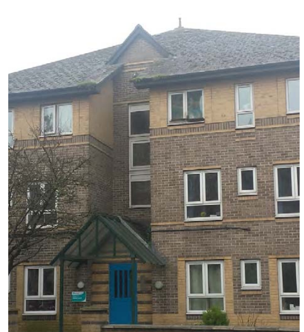
View of adjacent building brickwork and palette
