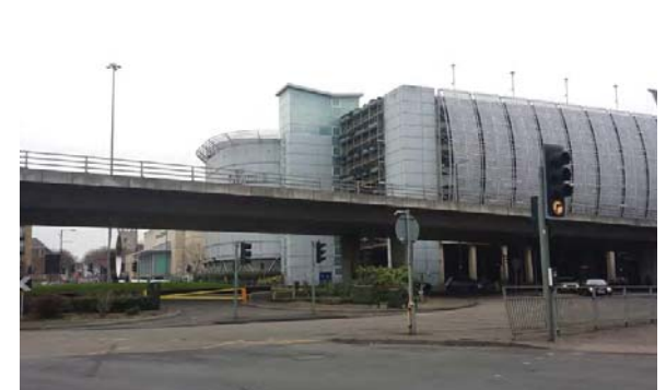
View from site to Reading town centre
