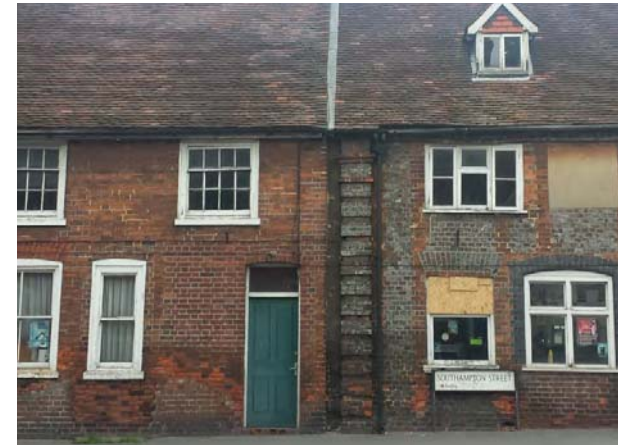
View of opposite buildings brickwork
