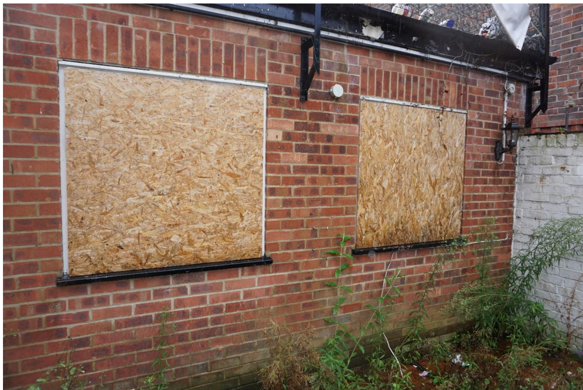
Photograph 4 – Single storey rear extension
