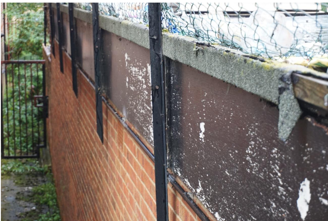
Photograph 10 – Change in level to the rear of the property
