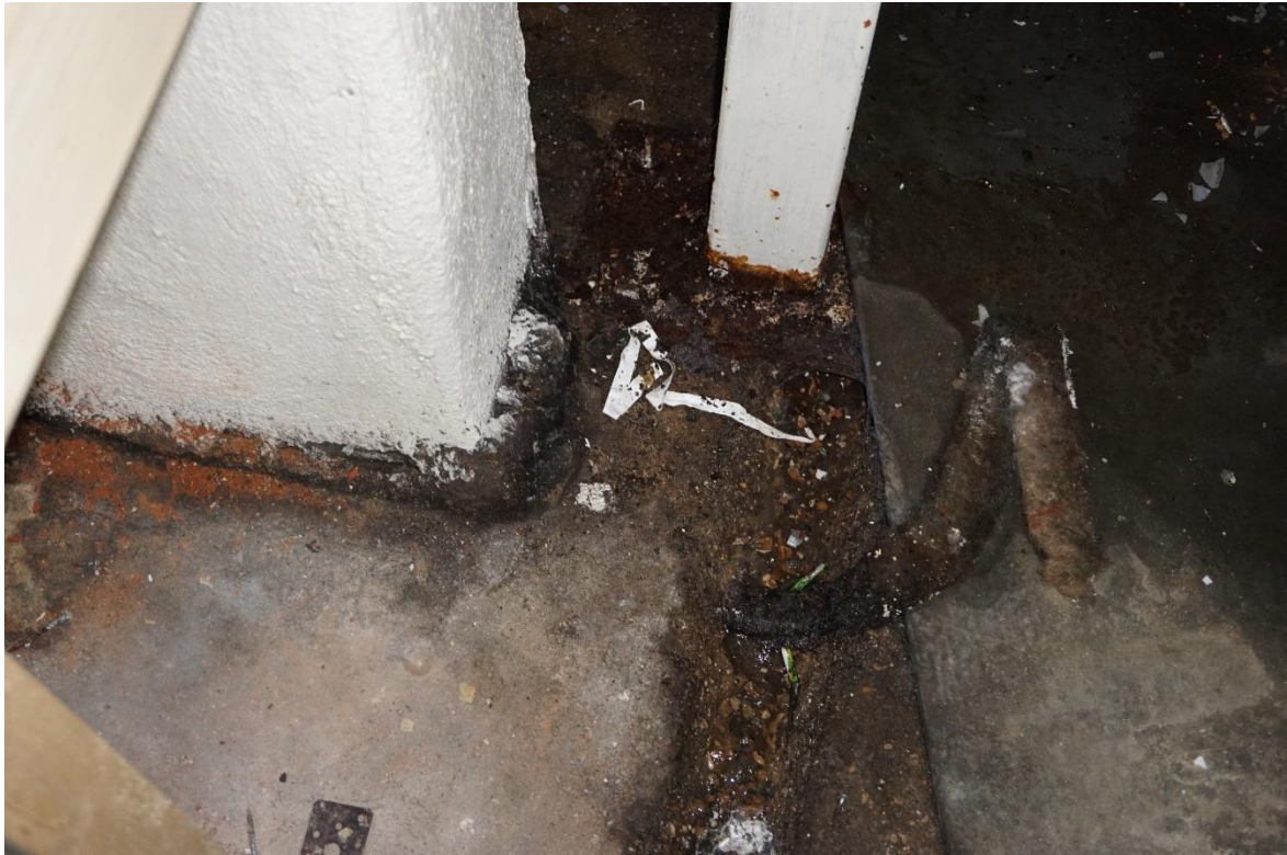
Photograph 16 – Corroded baseplate to goal posts
