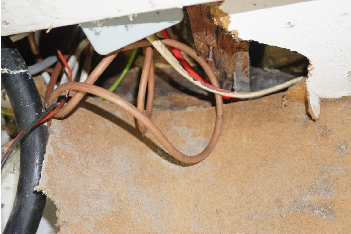
Photograph 13 – Decay to ground floor joists over basement
