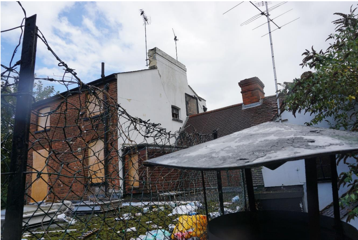
Photograph 3 – Rear and Left hang Gable
