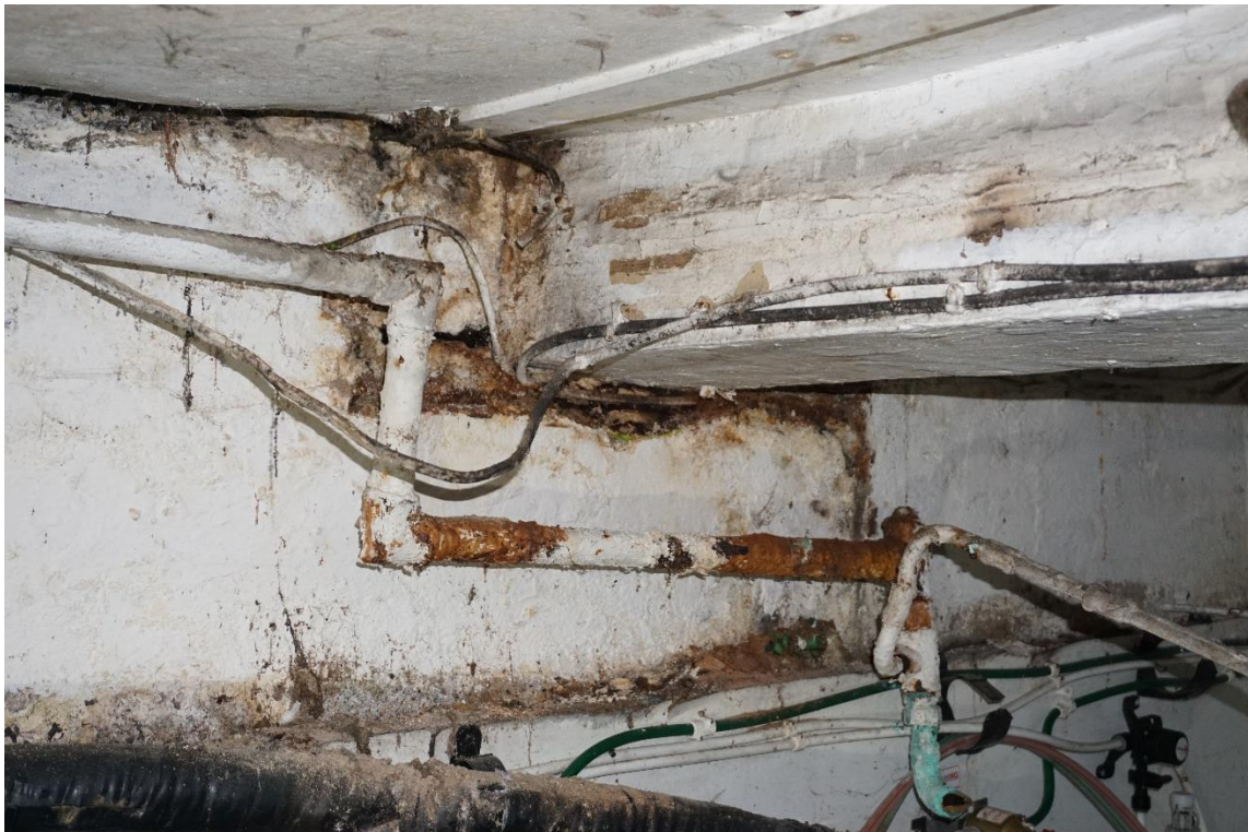
Photograph 14 – Decay to ground floor main beam at bearing
