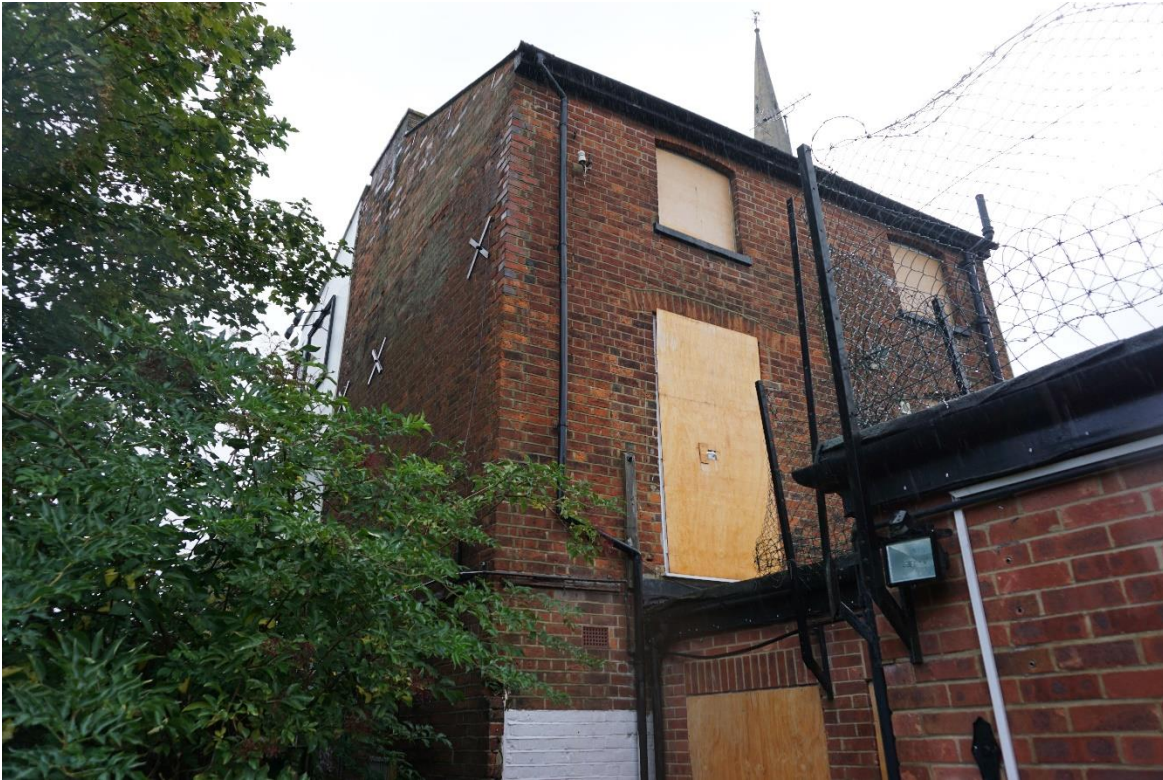
Photograph 2 - Rear & Right hang Gable
