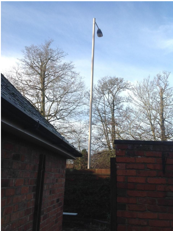
Street Lighting Column (Peppard Road) Located Outside the Boundary of the Staff Cottage (Viewed from Staff Cottage Grounds)
