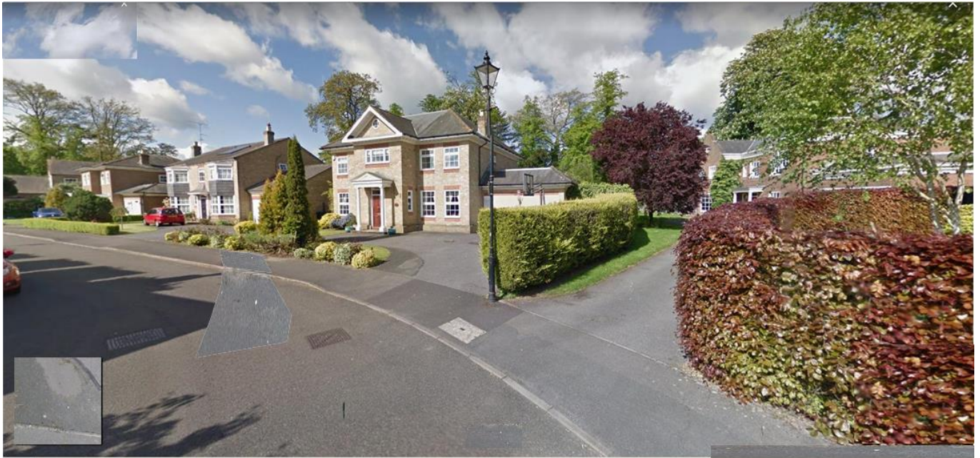
Image (3) OUTSIDE 8 DEVONSHIRE PK. VIEWING SOUTH WEST: SHOWS OPENNESS IN STREET SCENE AND PLOT INDIVIDUALITY
