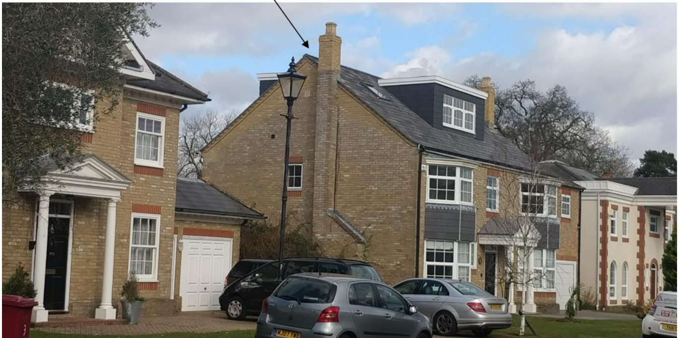
Image (4) 10 DEVONSHIRE PK.: – WITH RAISED RIDGE LINE & CHIMNEY STACK AND THE ONLY FRONT BOX DORMER ON THE CLOSE
