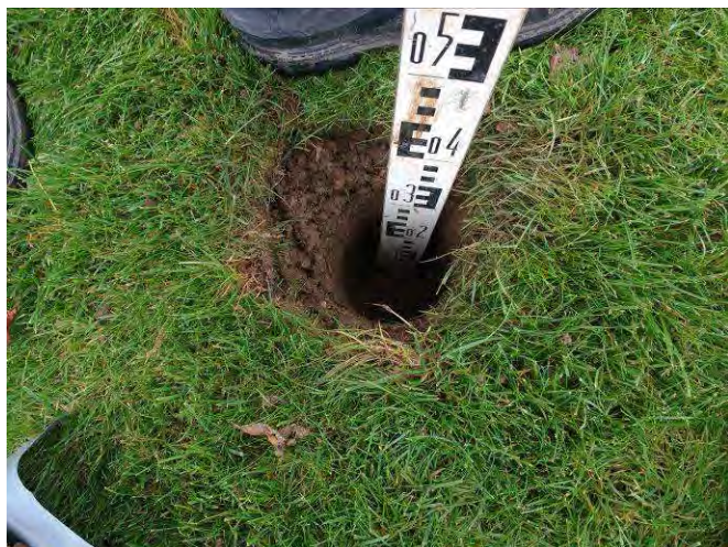
V5 _Communal soft landscaping area
