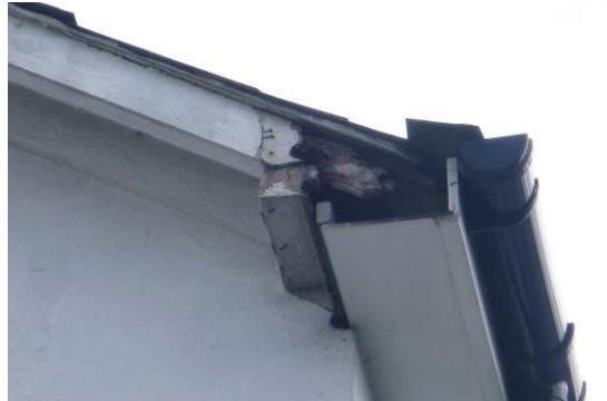
6. Open end of the soffit box.
