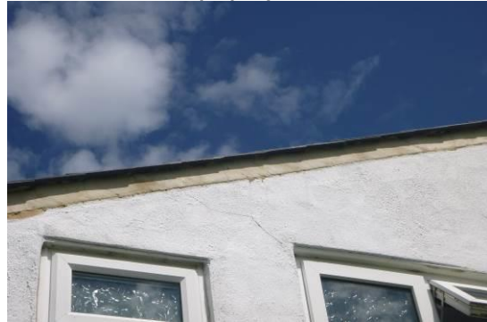
4. Sealed mortar at the verge of the rear extension.
