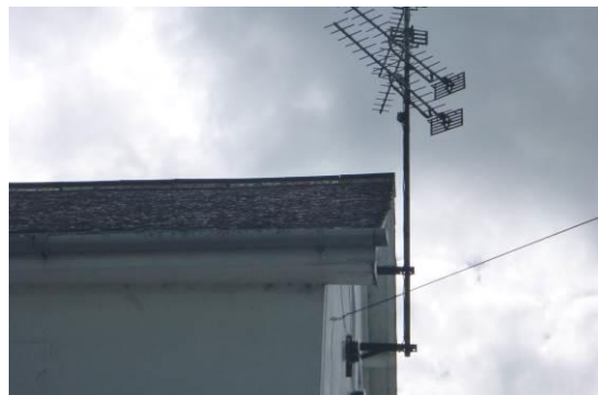
8. Tight soffit box at the front of the house.
