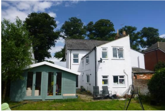
1. Rear view of the property.
