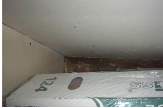
10. The plasterboard in the roof space.
