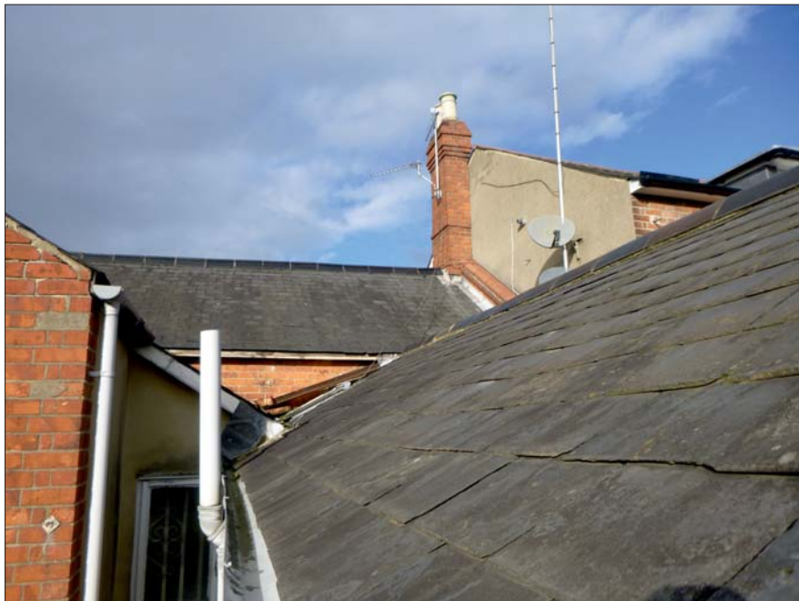
Photograph 3: Showing the roof inspected from the top of the flat roof extensions.
