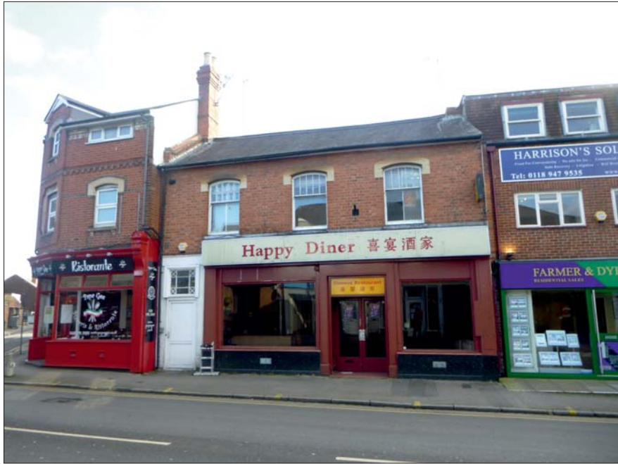
Photograph 1: Showing the building from the front of the site.
